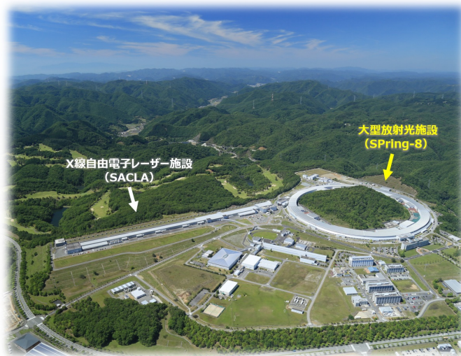
Figure 3.1: Aerial view of the SPring-8 .
