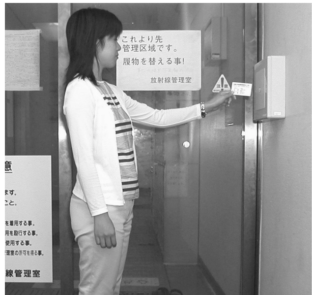
Fig.4 Card reader and the access door for the controlled area.
