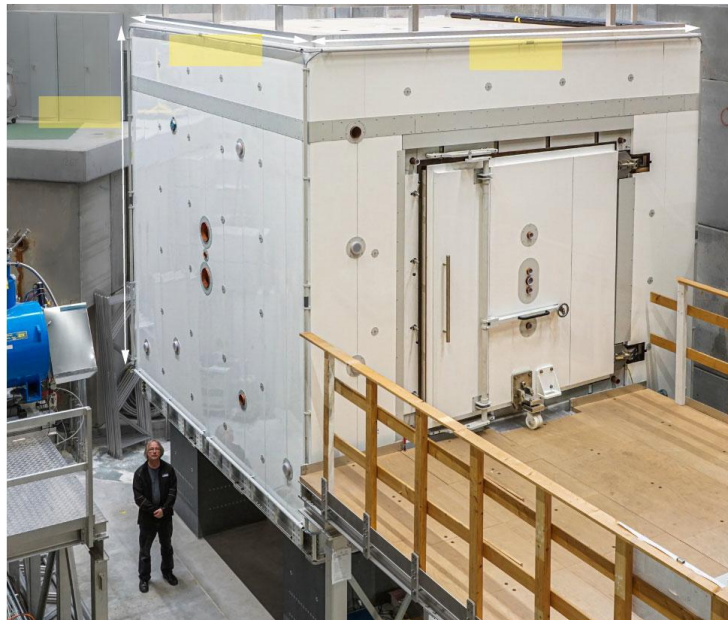
new Magnetic Shield Room
