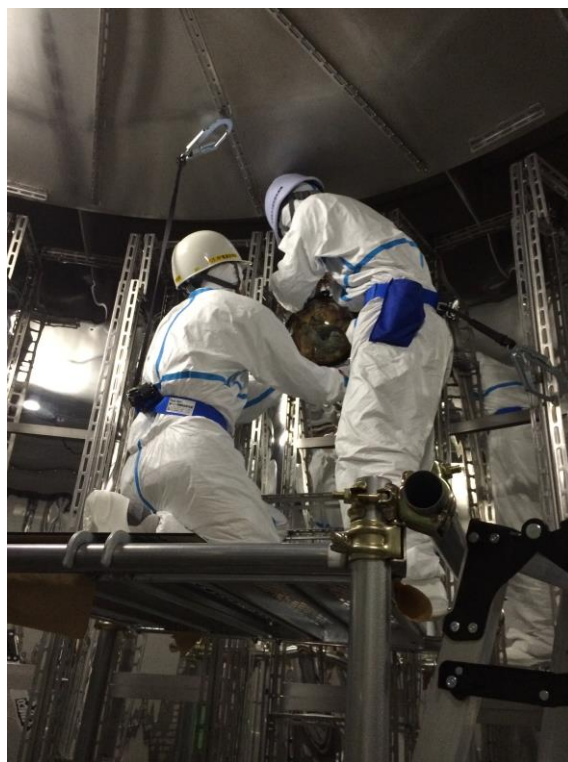
PMT installation
