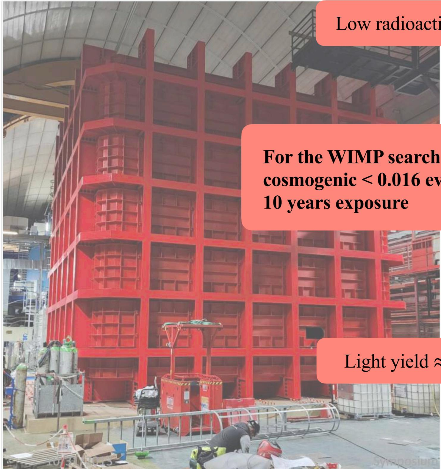
Low radioactivity membrane cryostat
