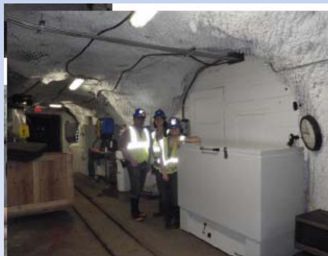
Underground detector storage
